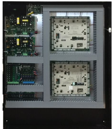
E8A - channel duct
